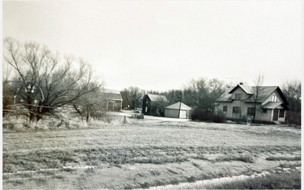
INTERSECTION WILLOWOOD DRIVE & HWY 13 (NW CORNER)
